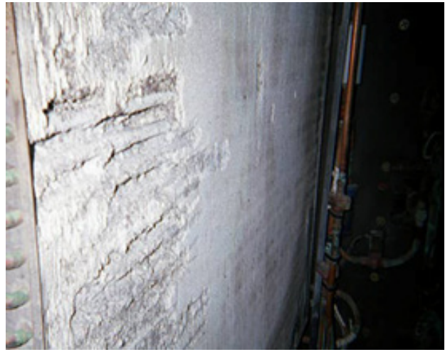
Corroded Dehumidifier
